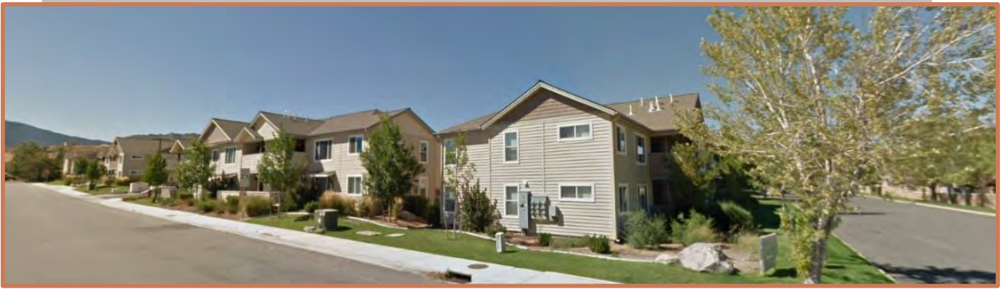
Photo: Summit Crest Apartments
